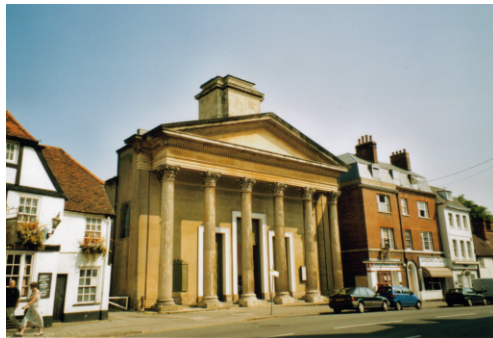
St.Mary's Episcopal Chapel, Castle Street
