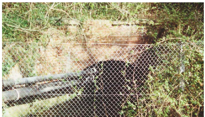
The small under-bridge over the Sul Brook
