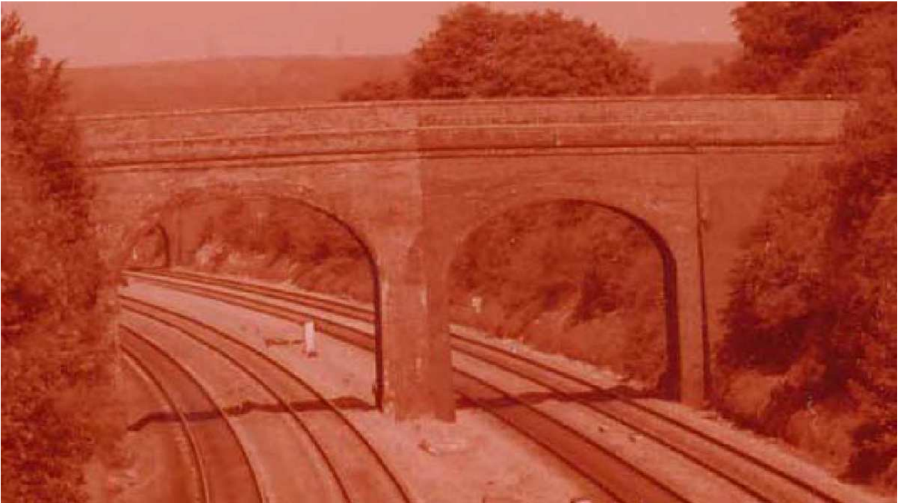
The Purley Lane bridge shows clearly the difference between the broad gauge arch (left) and the standard gauge one (right)
