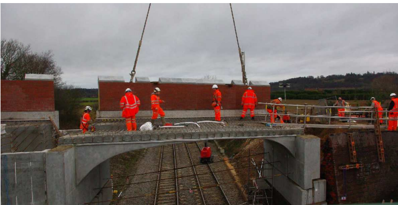
Rebuilding the Westbury Lane bridge lifting huge pre-built sections into place.
