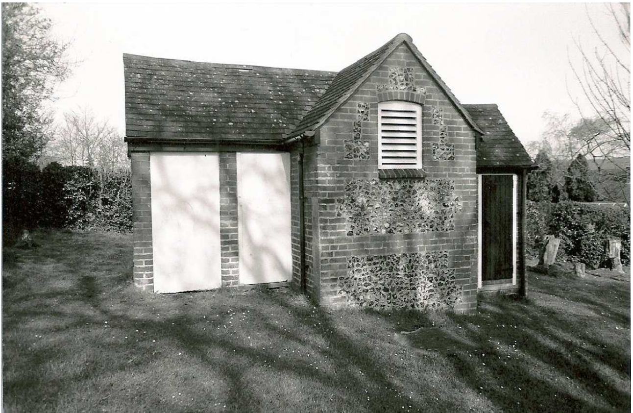
The old toilet block - long boarded up
