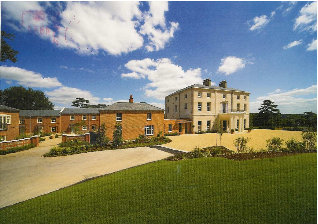
The result - flats and a courtyard
