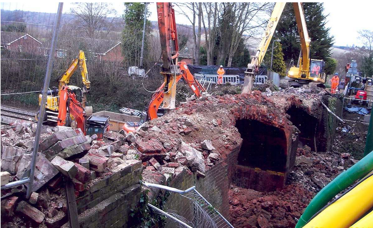
New Hill bridge being demolished
