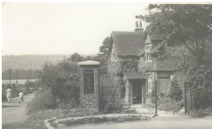
The Garden House as a Post Office
