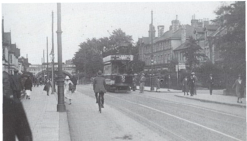
On Oxford Road - The Reading West Bridge is in the background [M080007]
