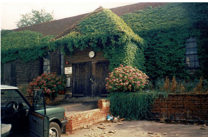
At Trenthams the barn was covered in ivy [M002216]
