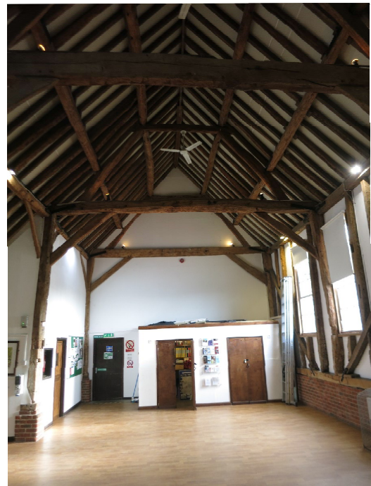
Interior of barn showing beam frames
