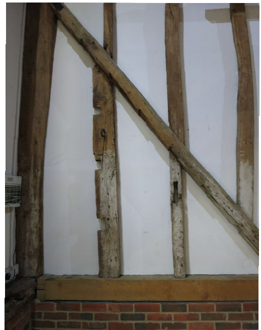
Timbers from the old manor house with original carpentry
