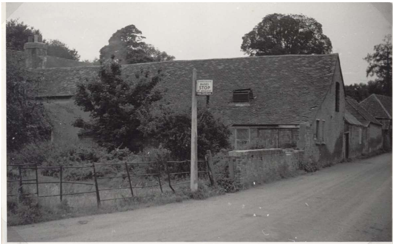
Home Farm, Purley in the 1960s - situated on The Street
