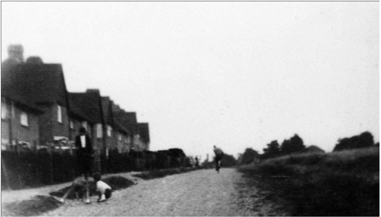
Glebe Road, Purley's first Council Houses
