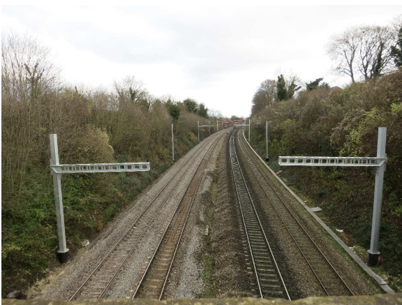
The first steps in erecting gantries for electrification
