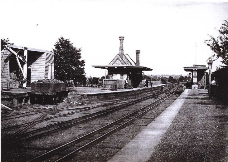
Pangbourne Station around 1860. The platform to the left has the ramp for loading coaches onto carriages.
