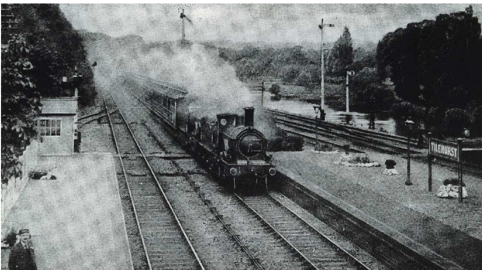
Tilehurst Station. You can see the short siding to the left which was used to hold the managing director's coach while he was at home. [M040000]
