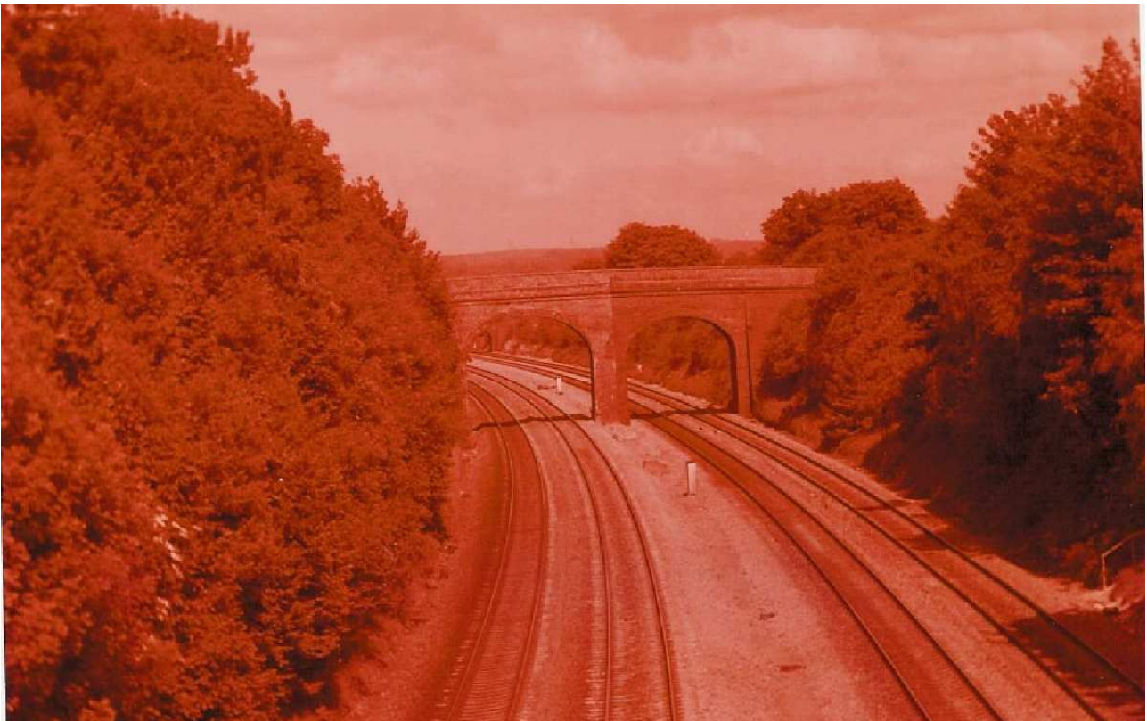
Purley Lane bridges - the arch on the left is the original Brunel arch for broad gauge trains and that on right for the widened (narrow) gauge lines.
