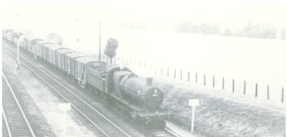
A 2800 class 2-8-0 on a mixed goods train near Westbury Lane [M]
