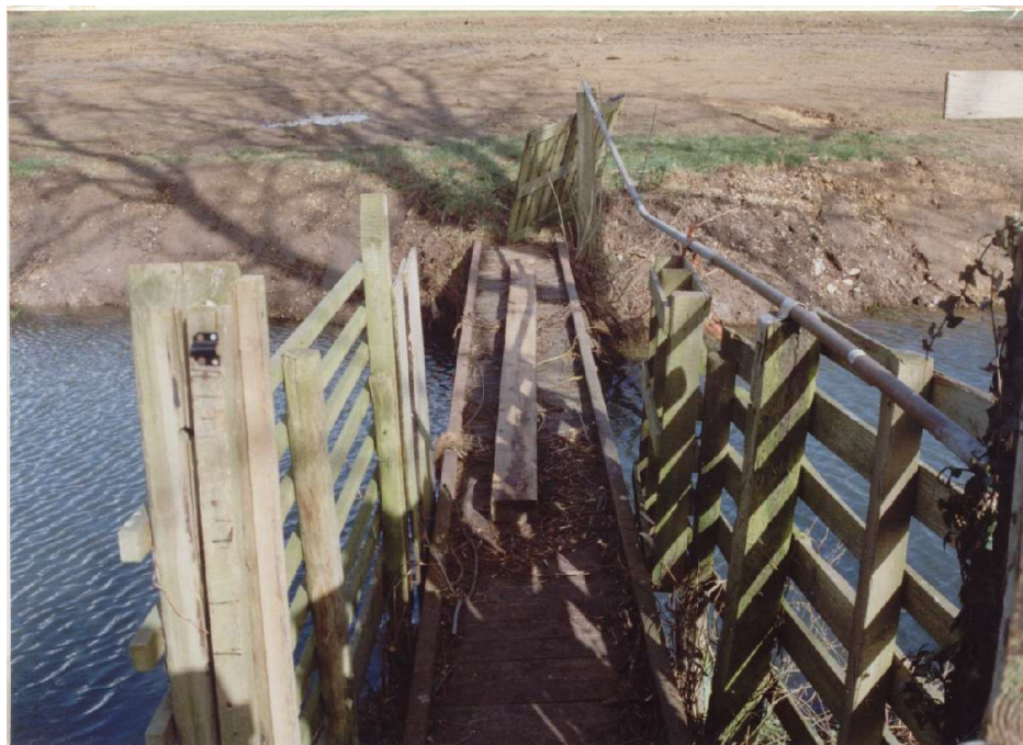
The bridge over the West Brook
