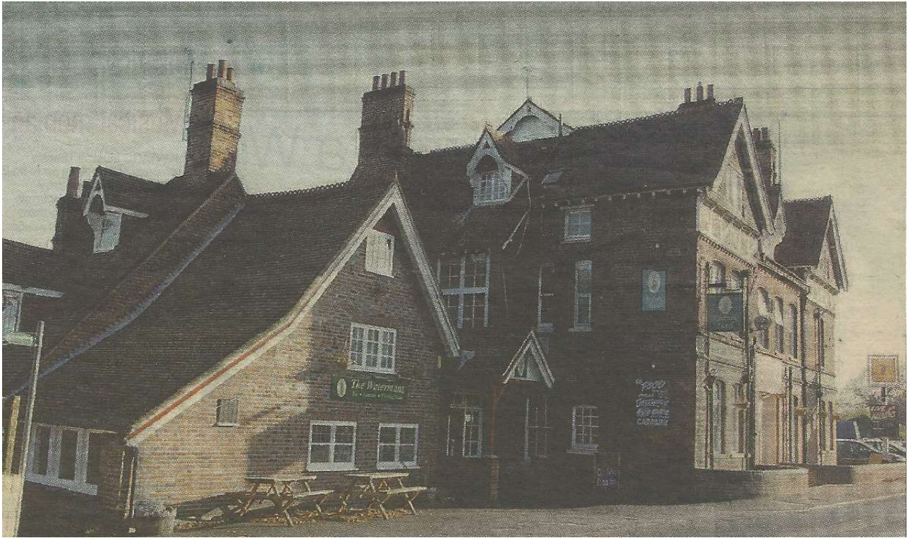
The west wing is the oldest part of the hotel [M001896]
